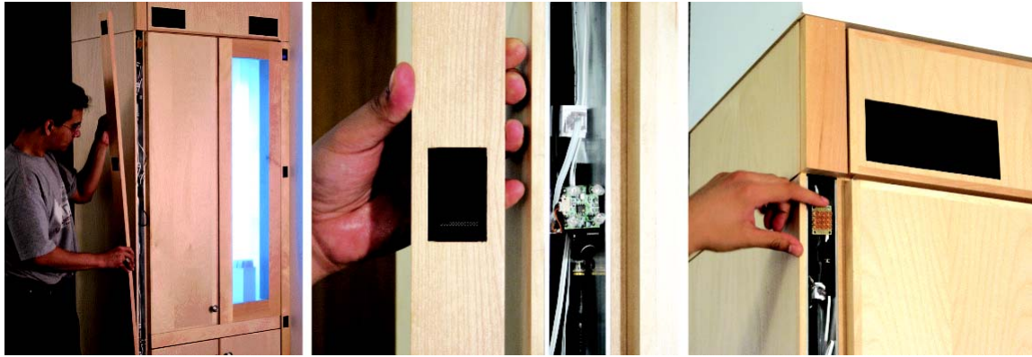
Fig 8 PlaceLab interior testing one aspect of Open Source Building — I3 components with sensing and addressable lighting infrastructure. Shown are hinged, accessible sensor bus raceways. All cabinets use the same embedded connections and technologies, simplifying installation and increasing flexibility. The facility contains hundreds of modular sensors.
